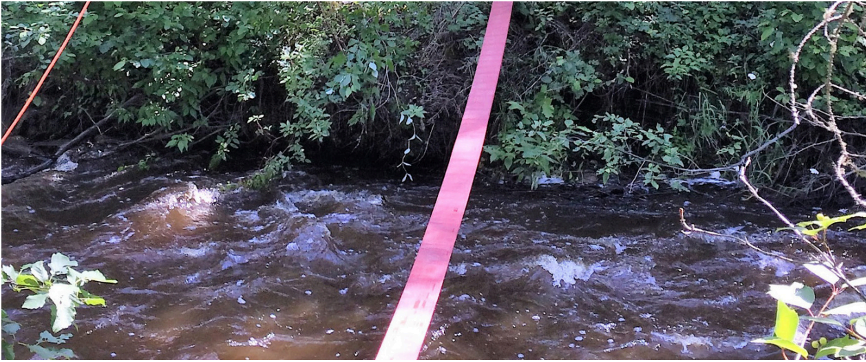
Safety Boss team used high angle rigs to move equipment up a hill and ensure we do not disturb the local creek or any nature in the process.
